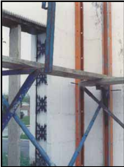
TEMPORARY HEADER BRACE
