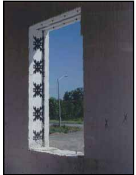
IF OVERSPAN, PLACE SPACER / WEB IN RSO AND REMOVE AFTER CONCRETE PLACEMENT
