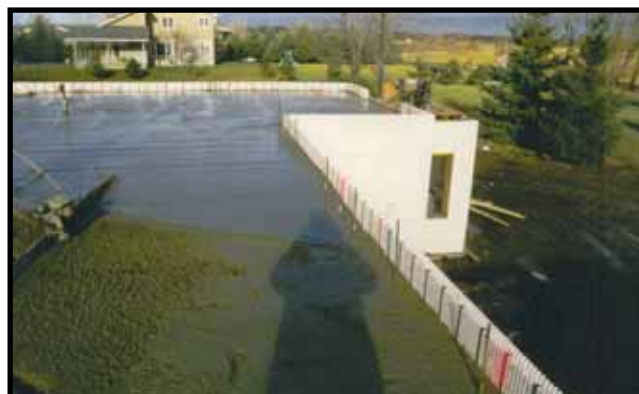
Hambro Concrete Placement
