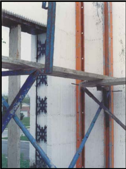
TEMPORARY HEADER BRACE
