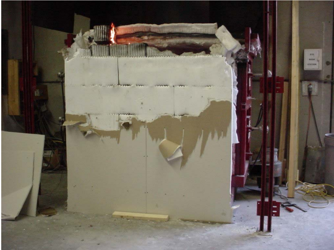
Unexposed Side After Fire Test, with Portions of Gypsum Wallboard Removed
