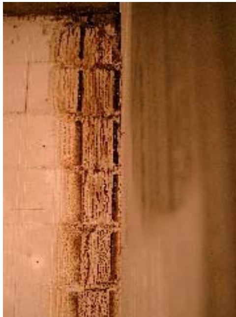
Test Sample After Removal of All Gypsum Wallboard, Left Wall
