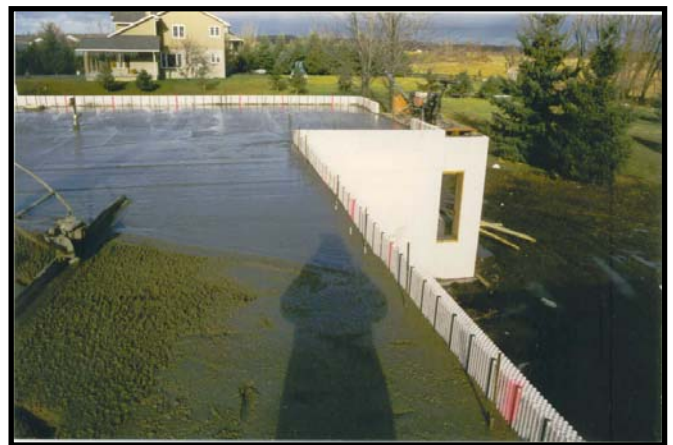
Hambro Concrete Placement
