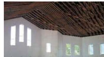
cut and carefully braced. Likewise, the unusual window openings and stepped sill plates required extra attention as well. According to the distributor who provided the ICFs, the church is extremely pleased with their new facility—including the ICF baptismal font. With 10,000 sq. ft of ICF walls, and only two trained installers on site, the church's walls are reportedly within an 1/8" of plumb, and the entire project was completed for around \$85 a sq. ft.
