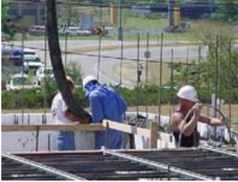
Work began in mid-March, and the walls went up fast. Workers were stacking walls on the fourth floor before the first floor foundation was completed. Trades (steel studding, mechanical, electrical, and plumbing) was "initiated or completed on the first three floors prior to placement of concrete on fourth floor," according to Buttrey.
