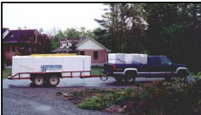
Shipment for 1200 ft 2 foundation, eight units high
