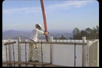
Concrete Placement
